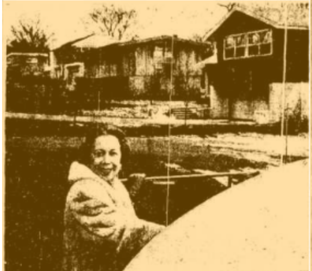
Houses with a design that is distinctively her own form a backdrop for Mrs. Lederer as she steps into her car to check on another of her many building projects.
