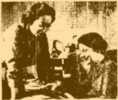
Greta Lederer, north shore builder, checks a construction detail with her secretary, Lucretia De Berry.
